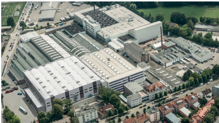
RENK AG, Augsburg Plant, corporate headquarters
